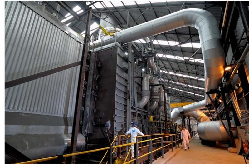
**Doosan Babcock OxyCoal Clean Combustion Test Facility. Image courtesy of Doosan Babcock**
