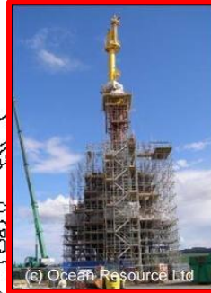
Sea Power Power Buoy North Sea
