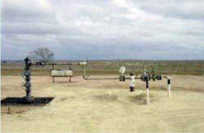
Well spacing is approximately 200m, with the wells generally arranged in a “5-spot” grid pattern (i.e. four wells in a square with a well in the centre).
