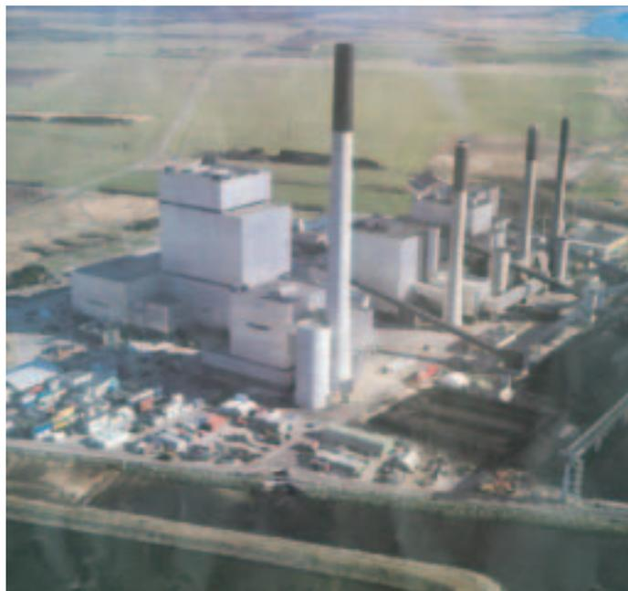
Alborg Unit 3 Double Reheat Supercritical Coal-Fired Plant at Vendsysselvaerket (courtesy ETSU)
