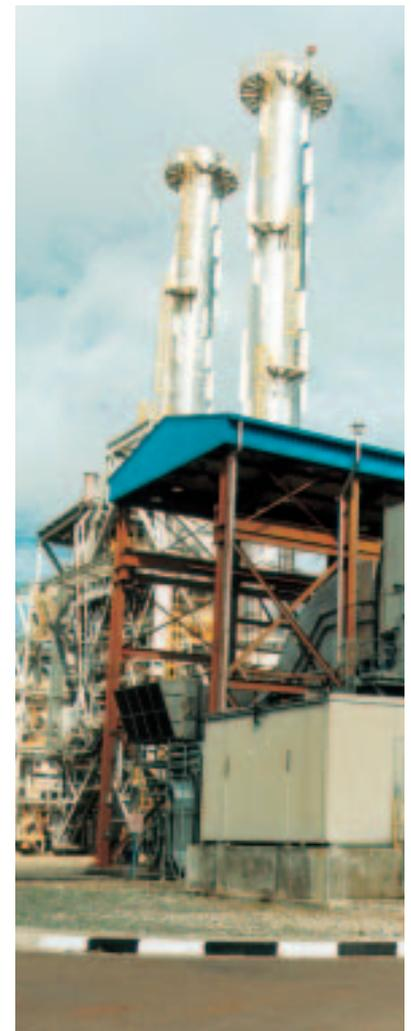
Two Industrial RB211s with Heat Recovery at Samarinda Power Station, Indonesia (courtesy Rolls-Royce)
